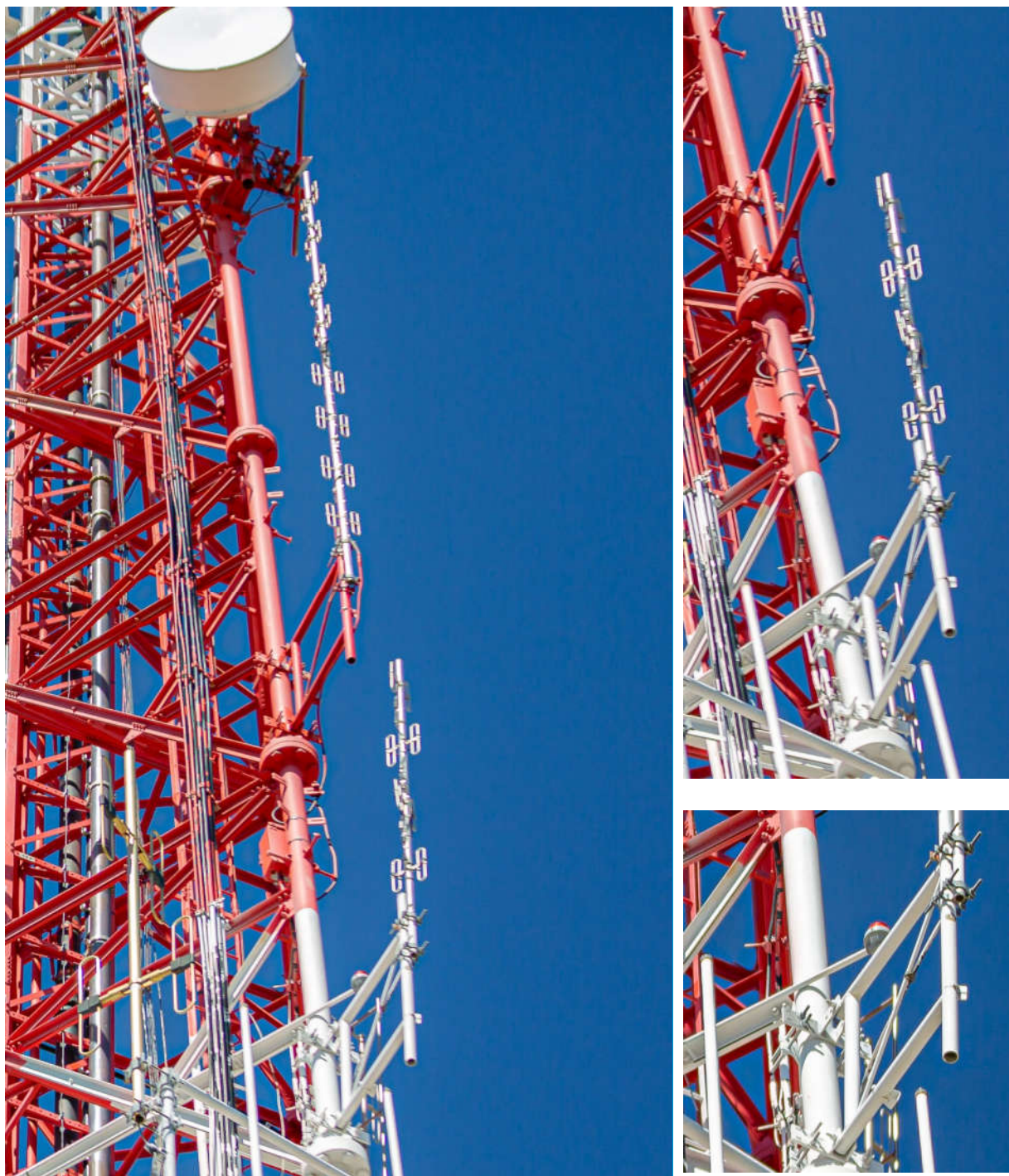
Figure 1-30 - NT-21 and NT-22 Mounts
