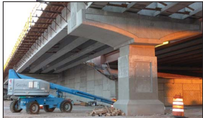
Above: Northbound direct connector at Bent 16 with girders at Montwood Drive.
