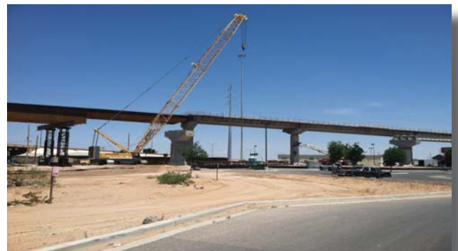
Above: Steel girder erection for the northbound direct connector.
