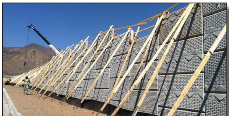
Below: MSE Walls under construction.
