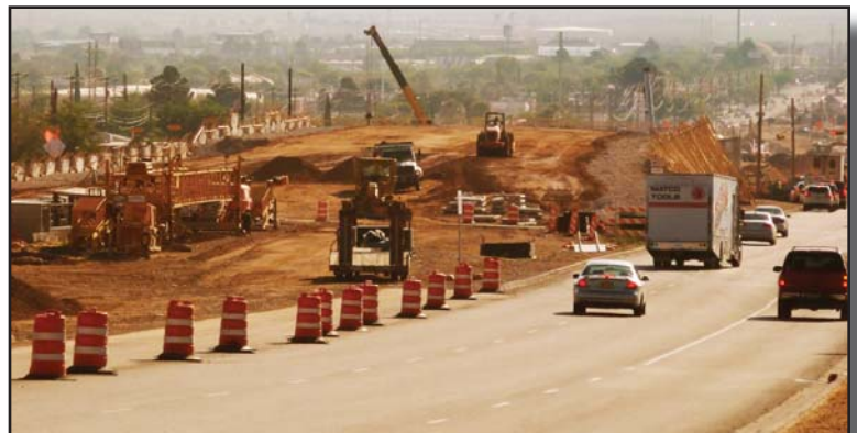
Above: Western embankment at the intersection of Kenworthy and LP375 mainlanes.
