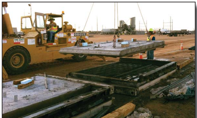
Below: MSE panels being removed from forms.
