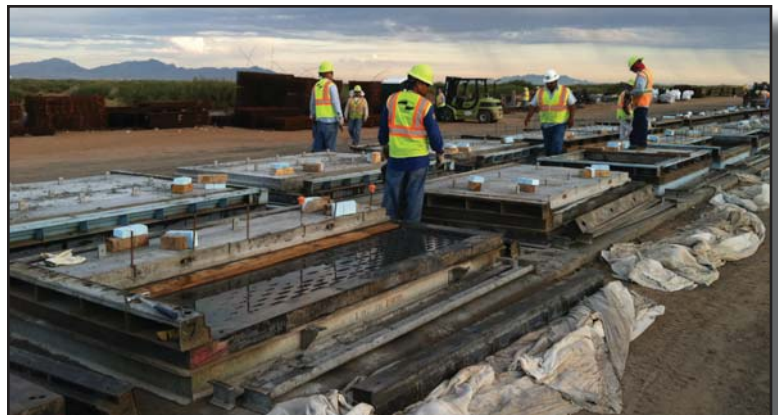
Above: MSE panels are inspected after curing for 24-hrs.
