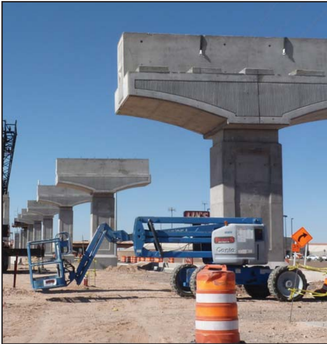
Above: Substructure for the southbound direct connector, as of mid-March, looking west.
